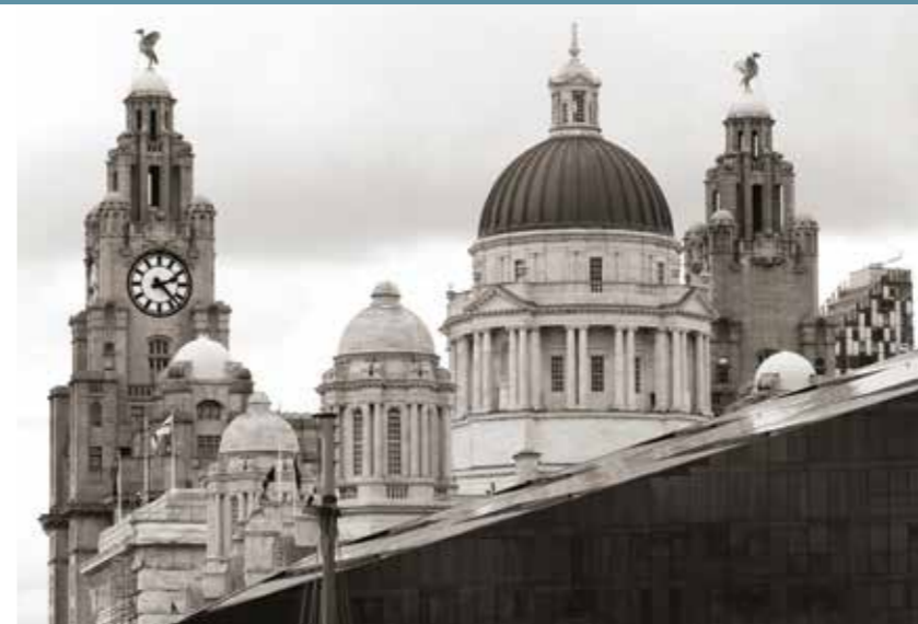
The 'Three Graces' of the world-famous Liverpool waterfront (from back to front): the Royal Liver Building, the Cunard Building and the former offices of the Mersey Docks and Harbour Board. iStockphoto / Thinkstock
