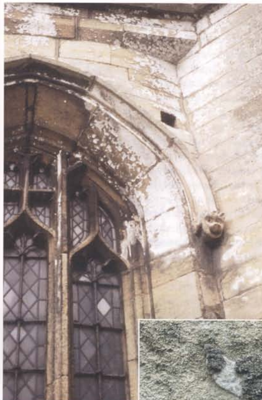
LEFT AND BELOW: Fig. 2. Window surround of a 14th century church at Fiskerton, Lincolnshire, showing extensive calcium oxalate encrustation. The inset shows a close-up of the encrustation demonstrating the role of D. massiliensis forma sorediata in its formation. COURTESY M.R.D. SEAWARD
