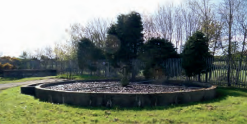
Trickling filter (TF) with traditional stone packing, typically used at small rural works. Mike Dempsey
