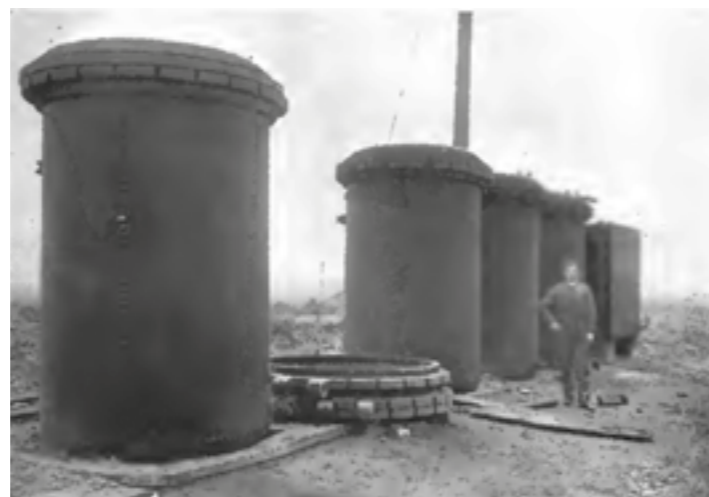
Fig. 2. Fermentation vats being erected at Synthetic Products Rainham, Essex during the Autumn of 1912. Martin, 1913
