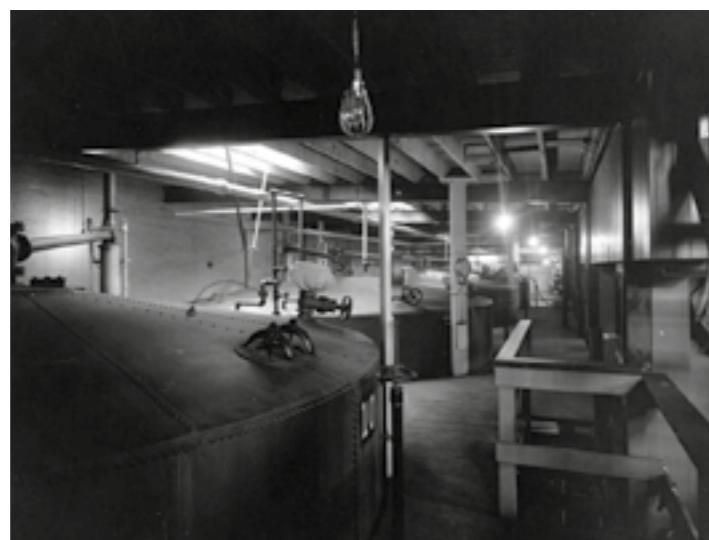
Fig. 3. Fermentors installed at British Acetone Toronto. Courtesy City of Toronto Archives
