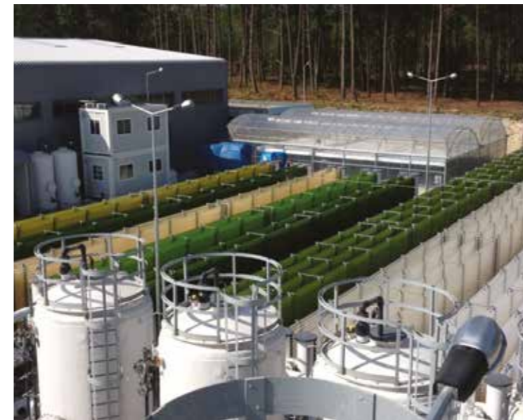
Fig 2. Algal growth facility (A4F-Algafuel SA, Portugal). This is a photograph of one of the largest algal growth facilities in Europe. The algal 'farm' was developed by A4F for Secil, a cement manufacturer sited nearby. The facility is powered by on-site generators with water supplied from a neighbouring quarry. Published with permission from A4F
