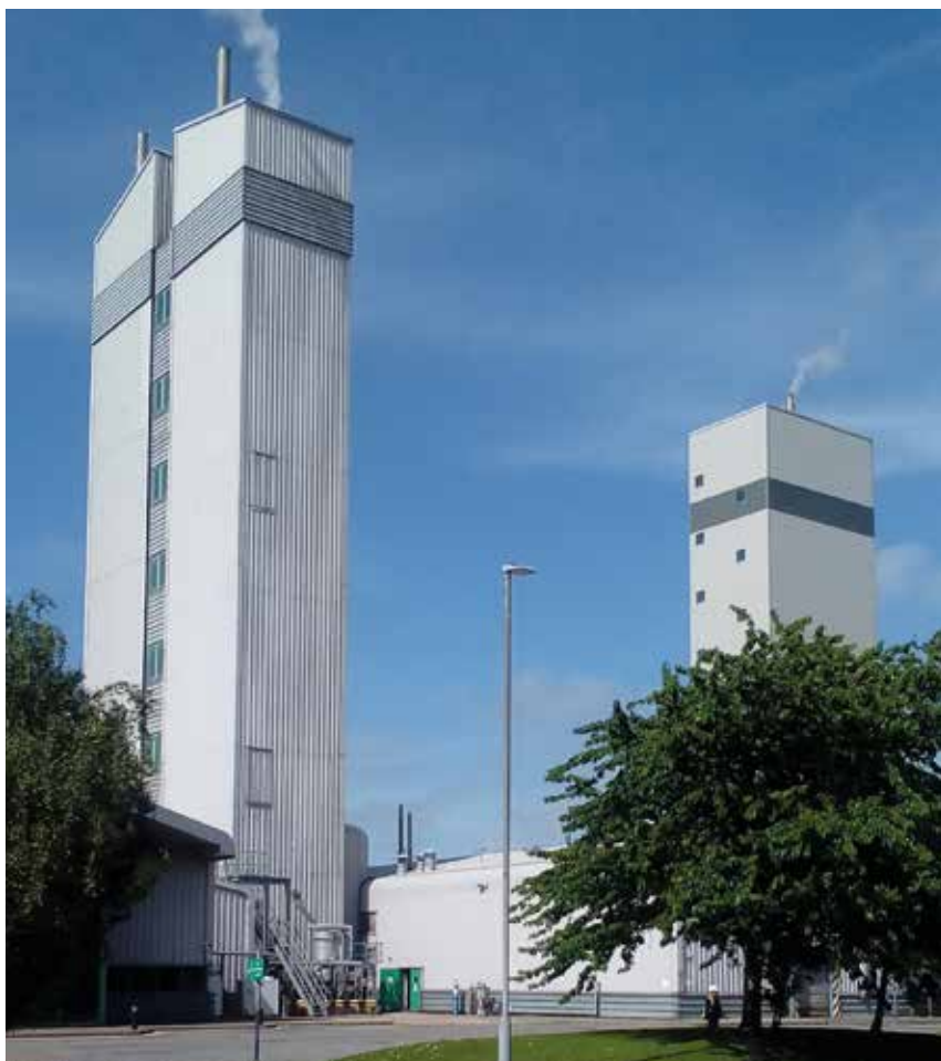
The towers containing the Quorn™ fermenters, two in the tower on the left and one in the right. Marlow Foods Ltd
